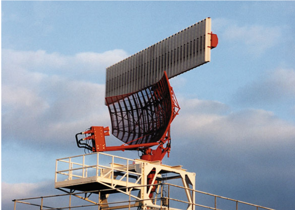
Figure 4: Primary and secondary co-mounted radar antennas
